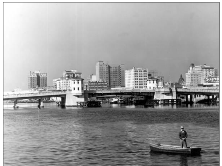
Platt Street Bridge in 1948 ( Image Courtesy FL State Archives )
